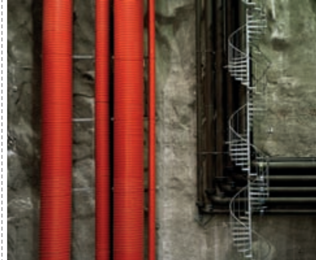
ONE OF THE MACHINE HALLS AT AURA POWER STATION.
