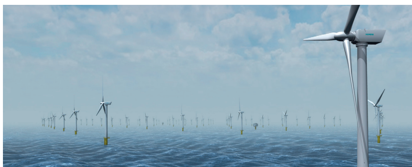
Sheringham Shoal Offshore Wind Farm, under construction off the coast of Norfolk in England.
