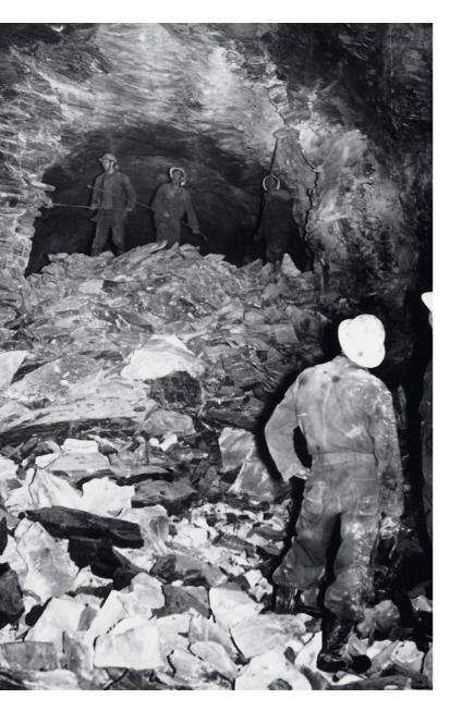
Blasting the inlet tunnel at Innset power station in Troms County. The state built Innset during the late 50s in order to support the electrification of the northernmost part of Norway, where electricity distribution was less advanced than in most other parts of the country.
