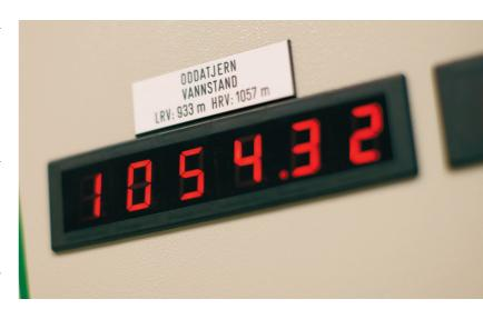
Statkraft has spent many decades on the research and development of electronic monitoring systems for the water levels in the company's numerous water reservoirs, which are spread all over the country. In the photo, the indicator at Oddatjern showing a near-maximal water level.
