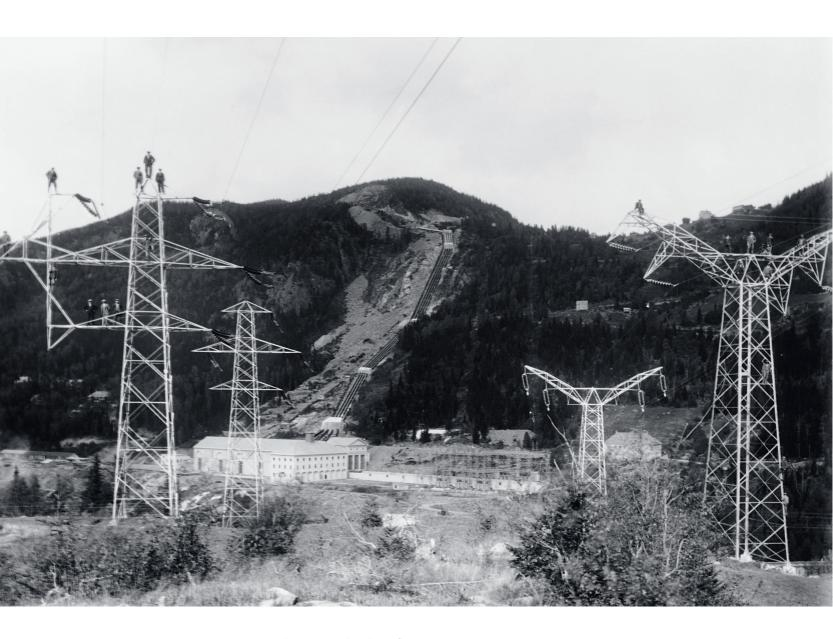
In central Østlandet, the Nore power station and its transmission lines made a major contribution to integration during the interwar years. Current from Nore started to flow in 1928 at a voltage of 132kV, the highest so far in use in Norway.
