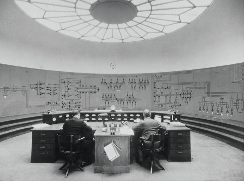
The central coordinating unit in Oslo, which started up in 1928. It coordinated generator outputs and exchange trade in power between the regional Østlandet companies. The centre was built and initially run jointly by agreement between the state and capital city's own electricity company. In 1932, the companies established their own organisation to manage coordination and called it Foreningen Samkjøringen (Coordination Board).
